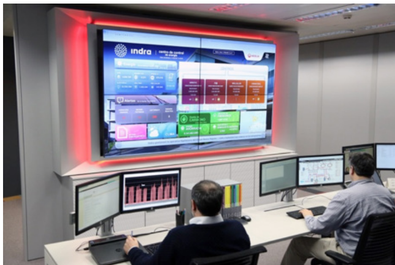
Energy control center at Indra's corporate headquarters
