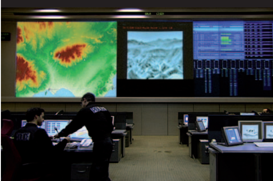
Command and Control Center
